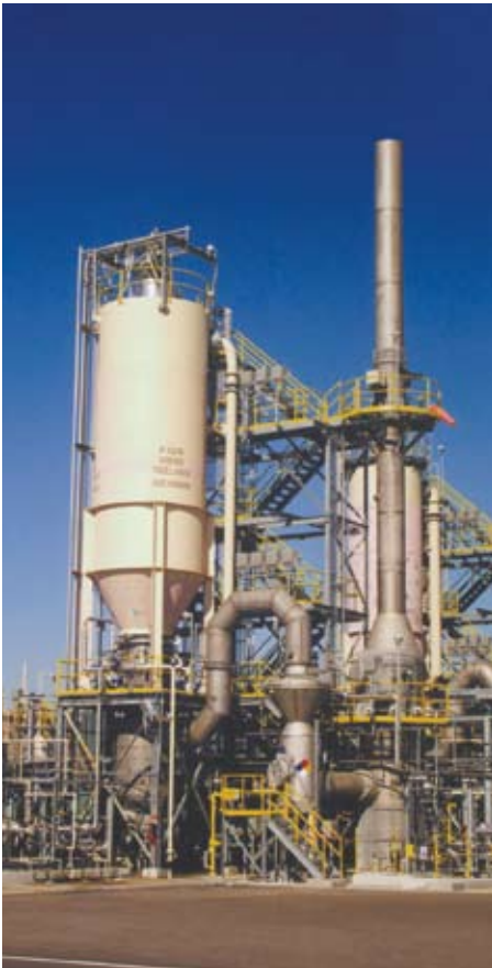
Down-Fired Thermal Oxidizer
