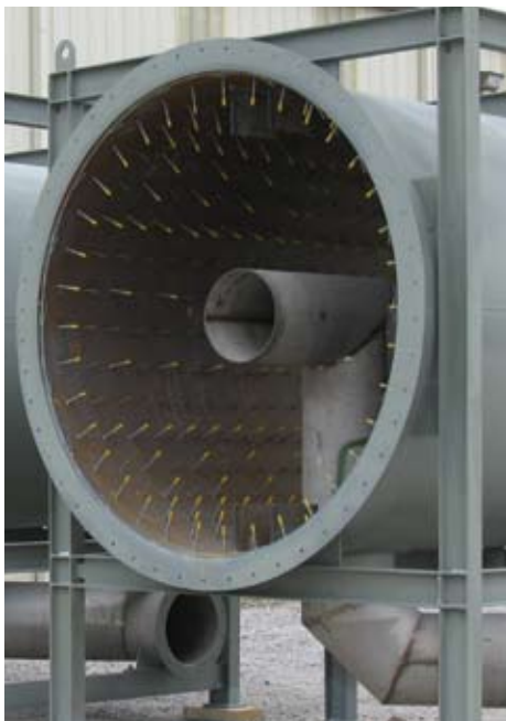
Inlet of SCR System
